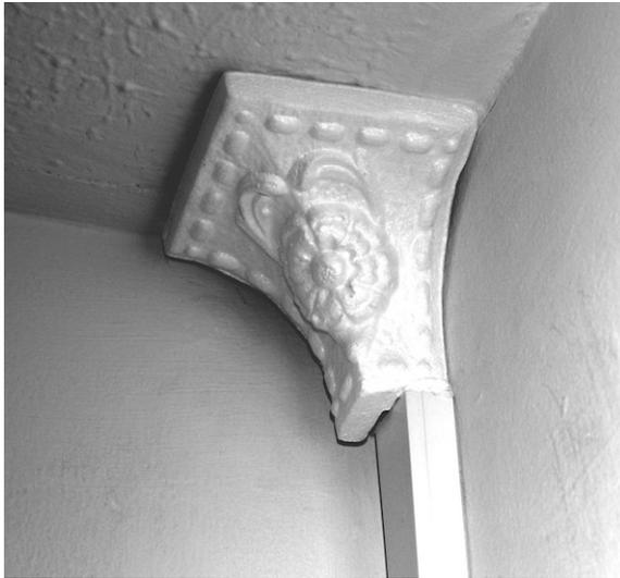
**Figure 4-1.** Trunking to hide the cables and a volute to (try to) hide the join.
