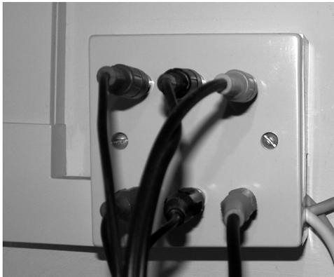
**Figure 4-3.** An AV connection for stereo and composite video. The top row sends the local AV signal upstairs, and the bottom row receives an AV signal to downstairs. Note the trunking on the left and the exit for network cables on the right, which is simply passed through from the trunking.
