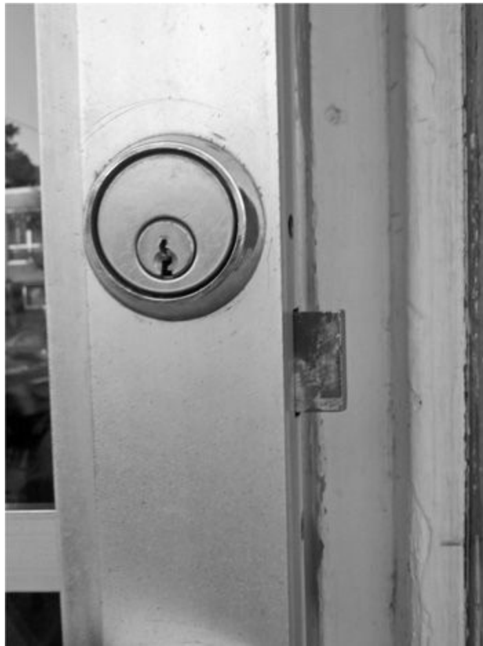
Figure 9-4 Deadbolt-type straight plunger
