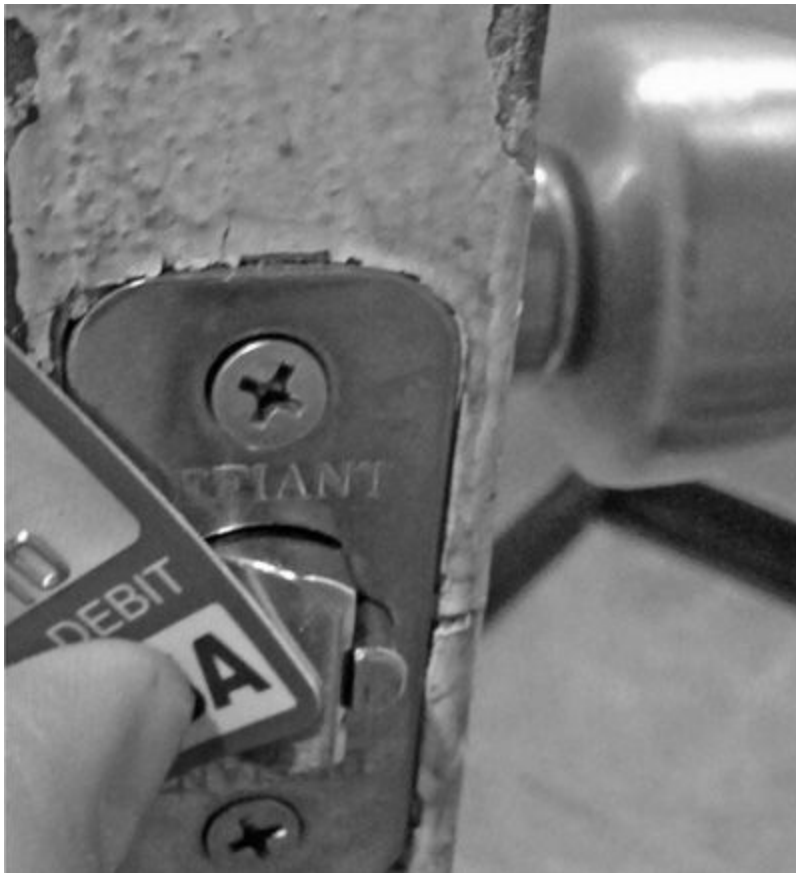
Figure 9-13 Shimming lock plunger with credit card
