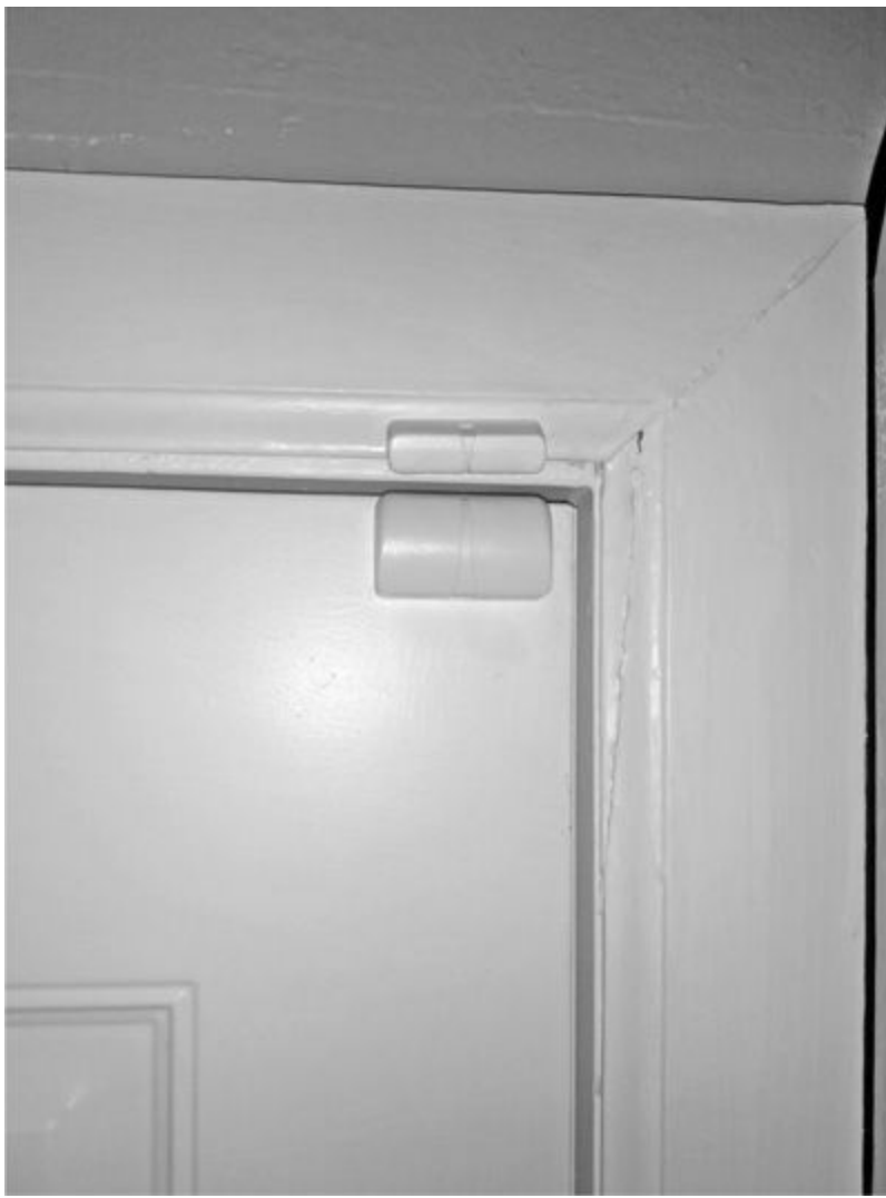
Figure 9-27 Magnetic contact switch
