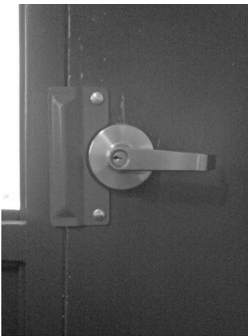
Figure 9-14 Shim guard blocking access to plunger
