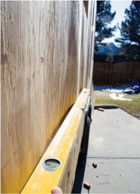
Warped Sheathing
