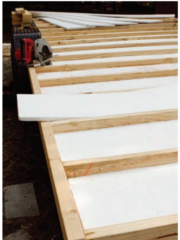
Subfloor Insulation
