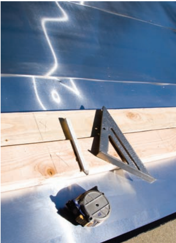
Top Plate and Kick Plate Marked
