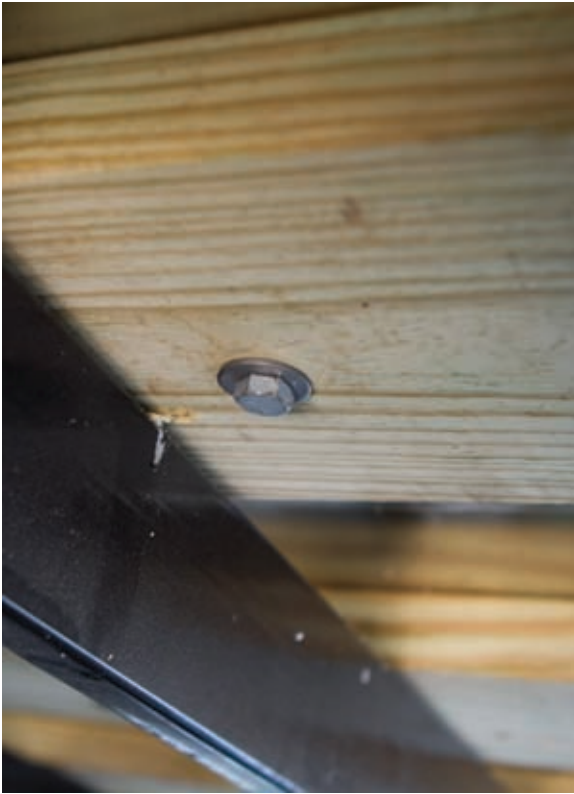
Lag Screw Under Trailer
