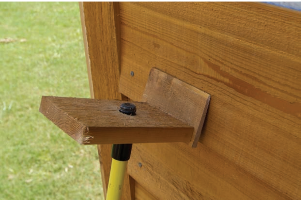
Hand Made Tool to Help Install Siding
