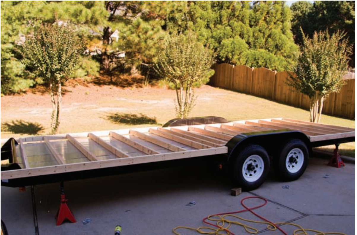
Subfloor Framing Attached to Trailer
