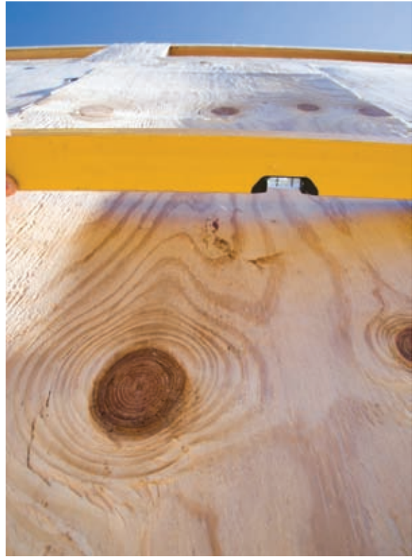
Warped Sheathing
