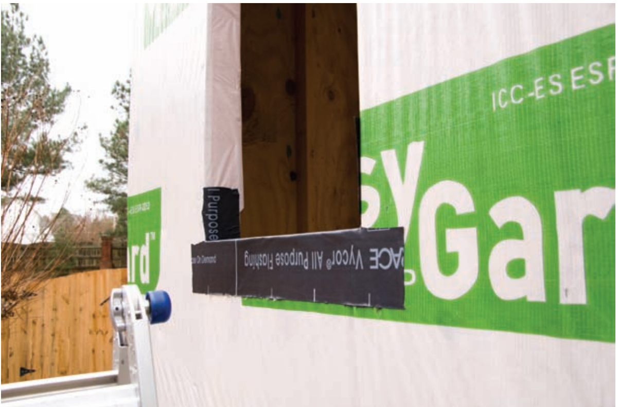
Flashing Attached to Sill Plate
