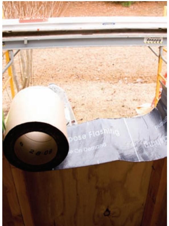
Flexible Flashing Laid Out
