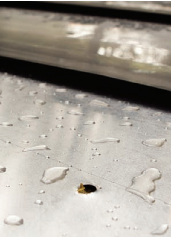
Pre-Drilled Hole in Trailer Decking
