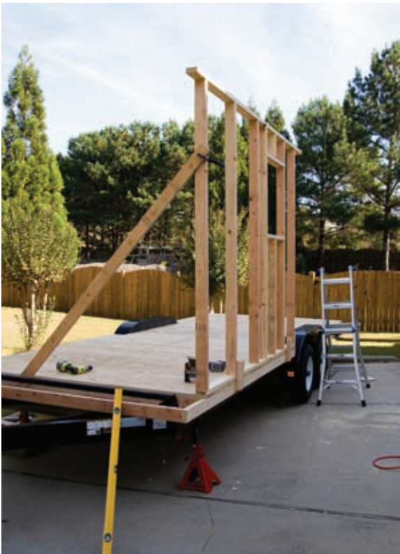
Wall Stood Up and Braced
