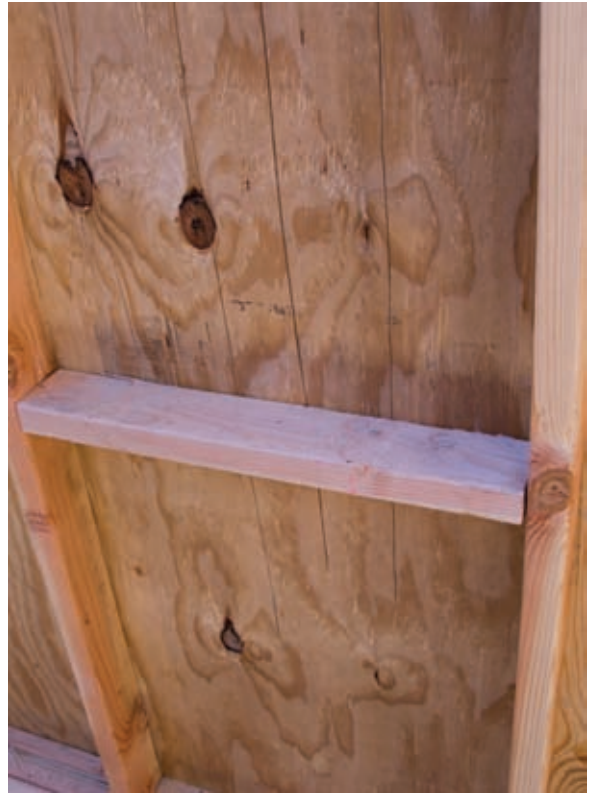
Wall Braced on the Inside
