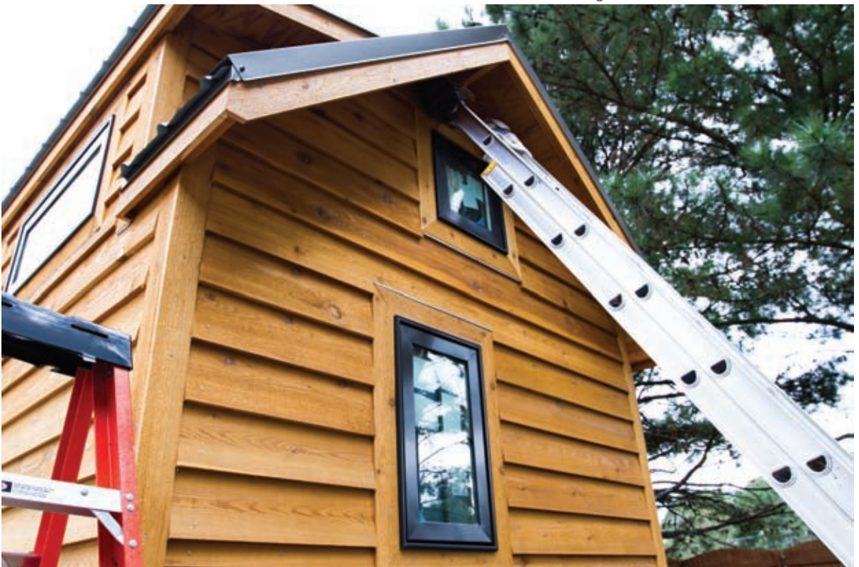
Siding Installed on Gable End
