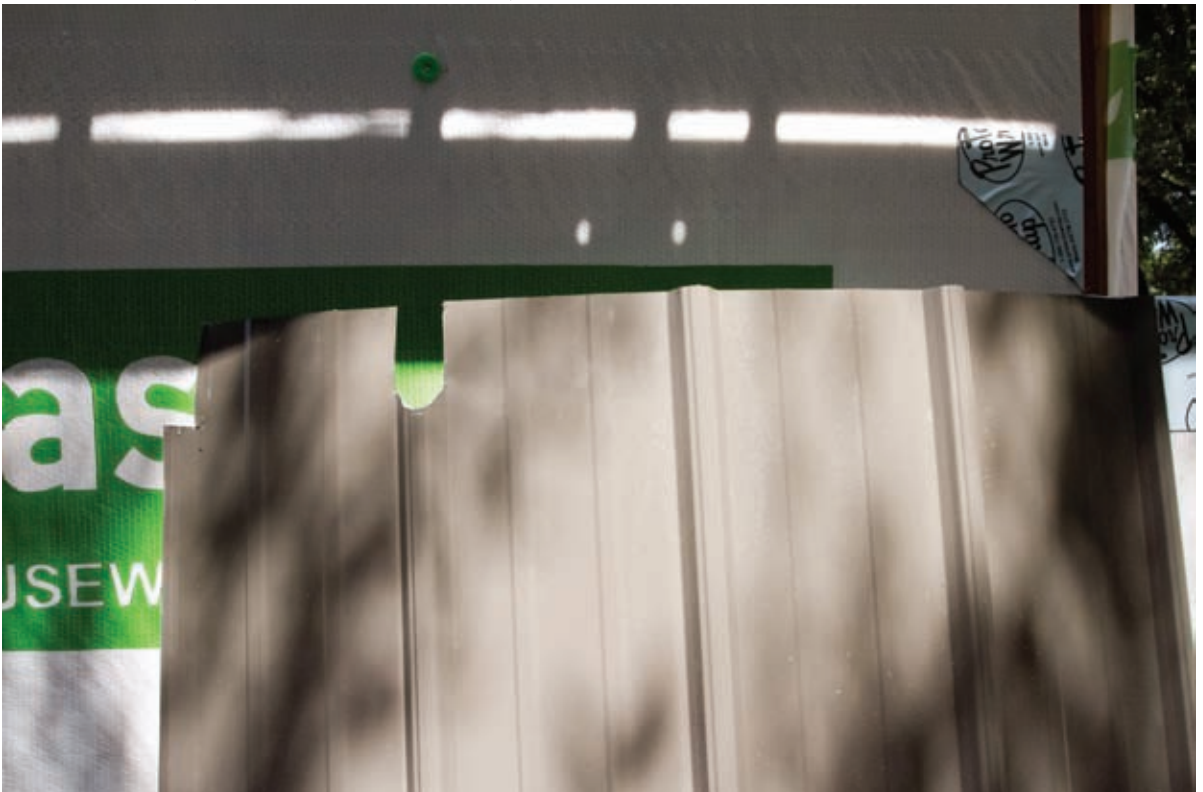
Roof Panel Trimmed to Fit
