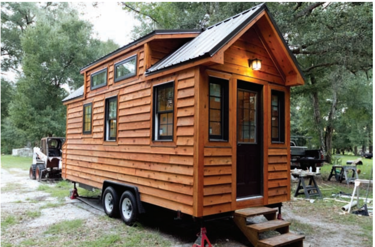
Trim and Siding Completed
