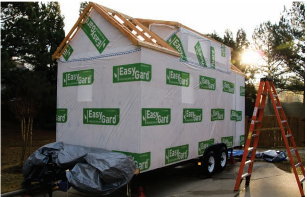
House Wrap Installed
