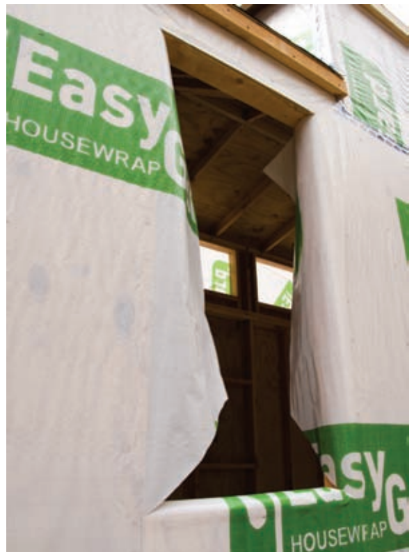
House Wrap Cut for Window
