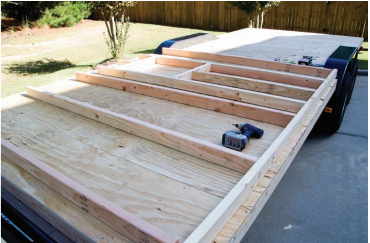
Wall Partially Completed
