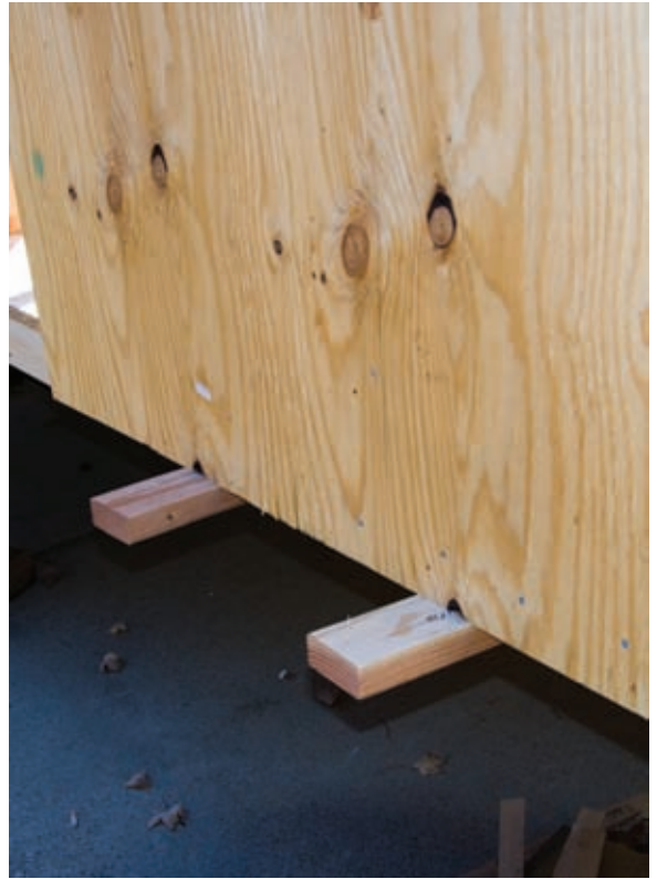
Temporary Bracing Under Subfloor
