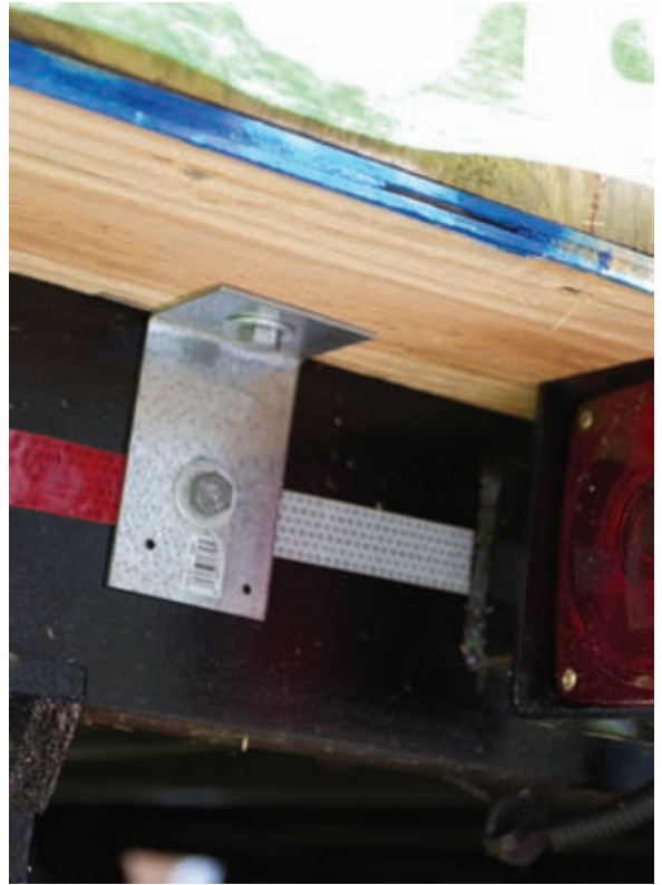
Bracket Attaching Subfloor Framing to the Trailer
