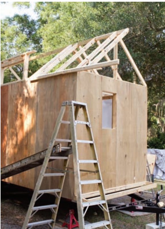
Rafters Being Installed
