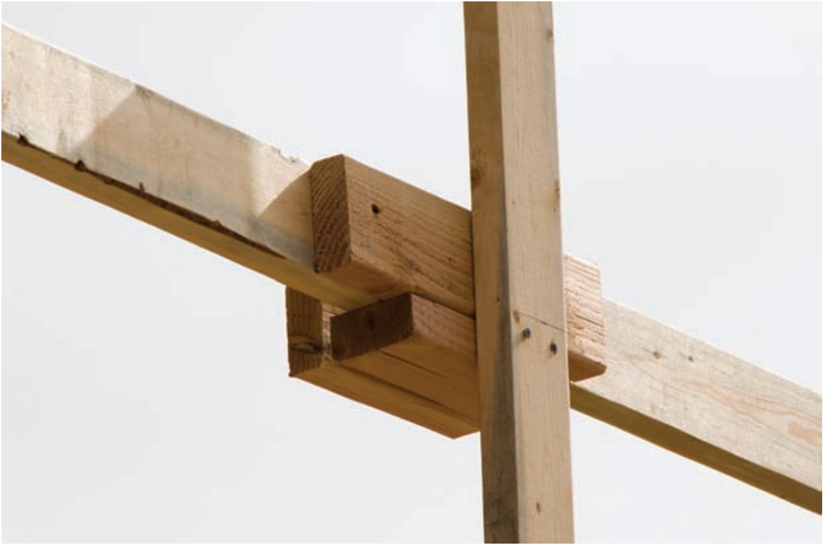
Temporary Support for Ridge Beam
