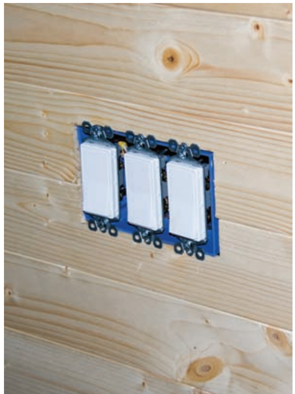
Siding Around Switch
