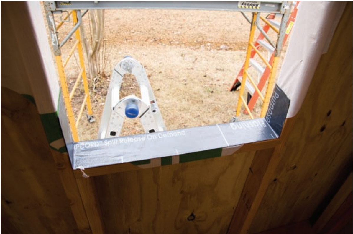
Flashing Attached to Sill Plate
