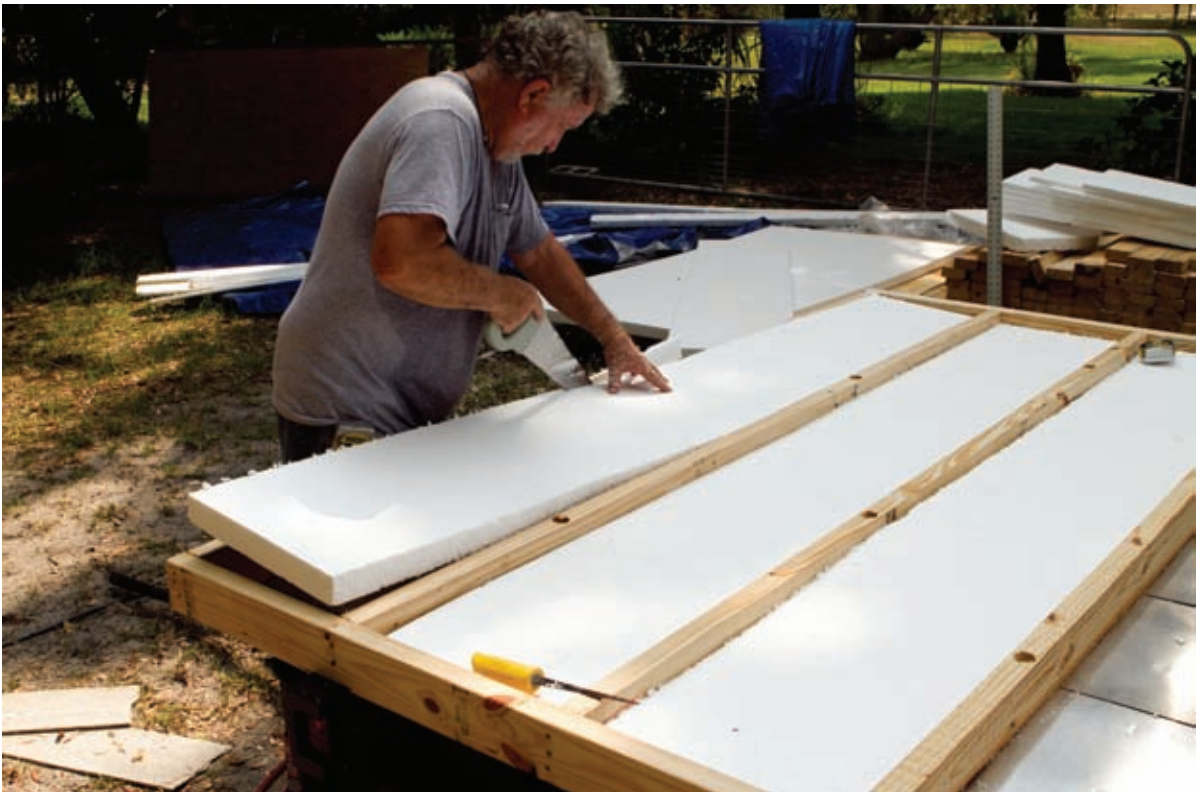
Subfloor Insulation Being Installed
