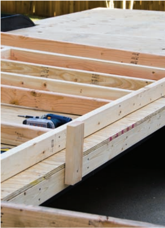
Temporary Bracing at Subfloor Edge
