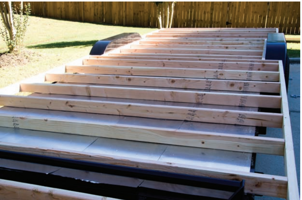
Subfloor Framing Completed
