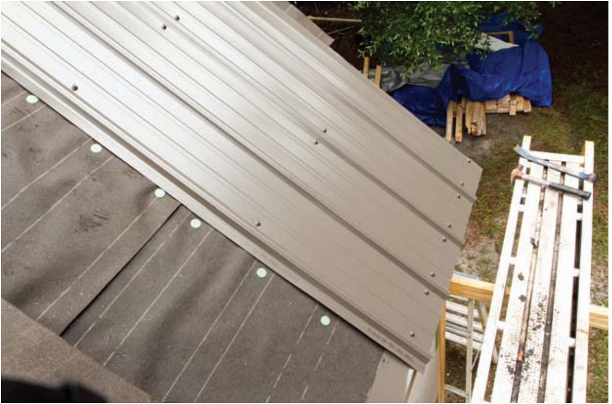
Installed Roof Panel
