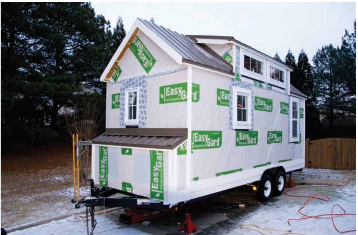
Trim Installed and Starting on the Siding
