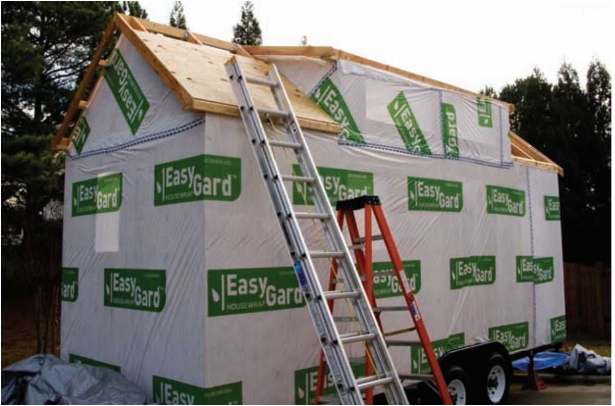
Roof Sheathing In Place
