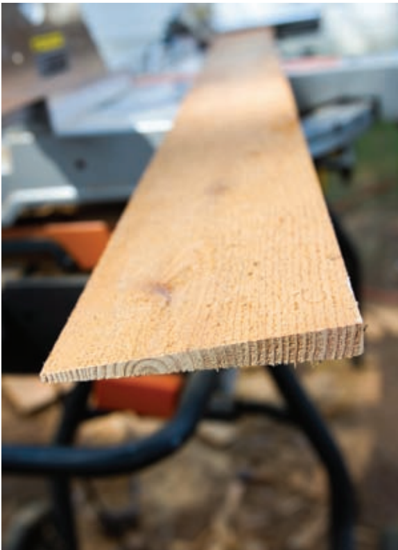
Cut Siding for Window Sill
