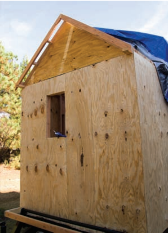
End Wall Sheathed
