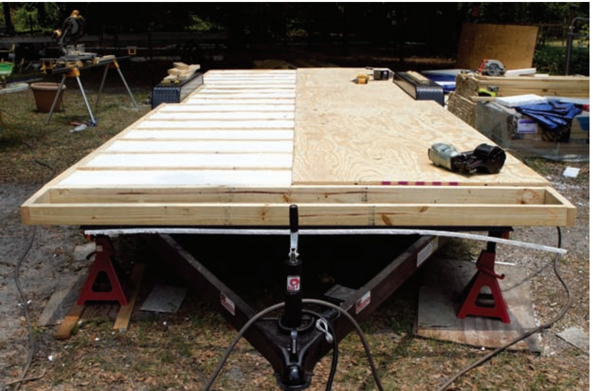
Subfloor Sheathing Half Installed
