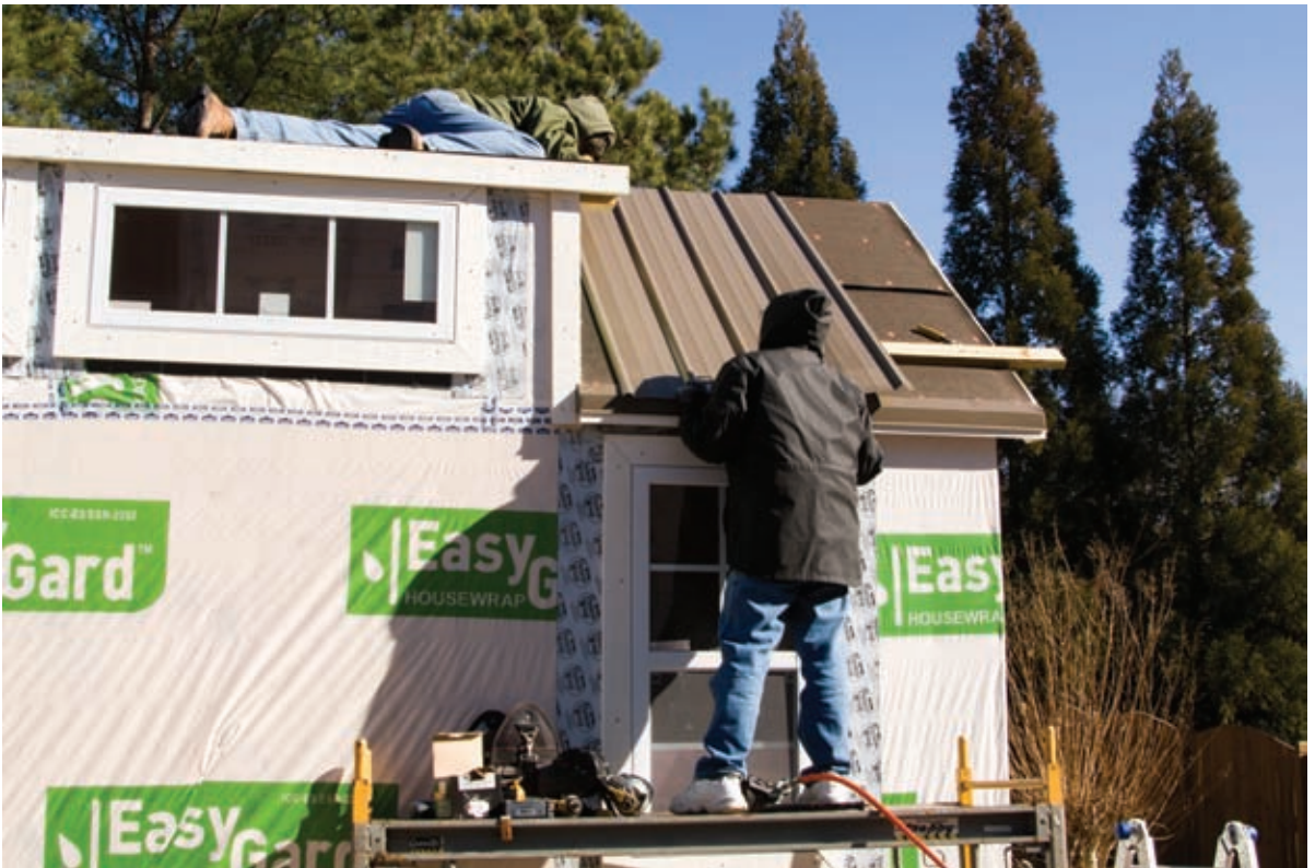
Roof Panel Being Installed
