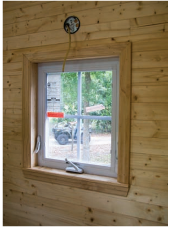
Trim Around Kitchen Window
