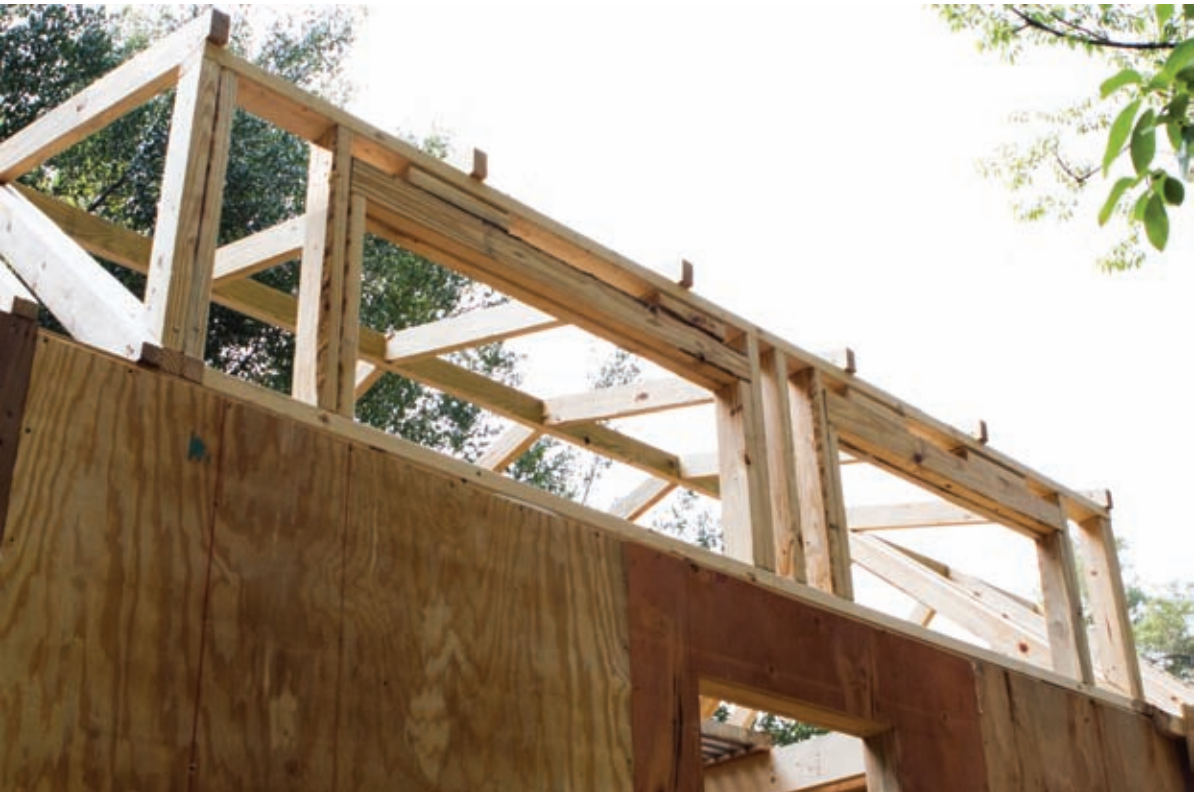
Upper Wall Section Assembled
