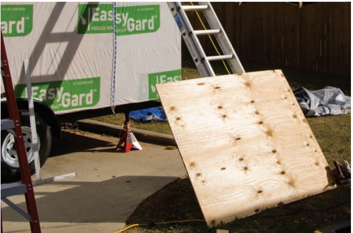
Roof Sheathing Ready to be Slid In Place
