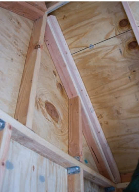
Deadwood Installed in Ceiling Corner
