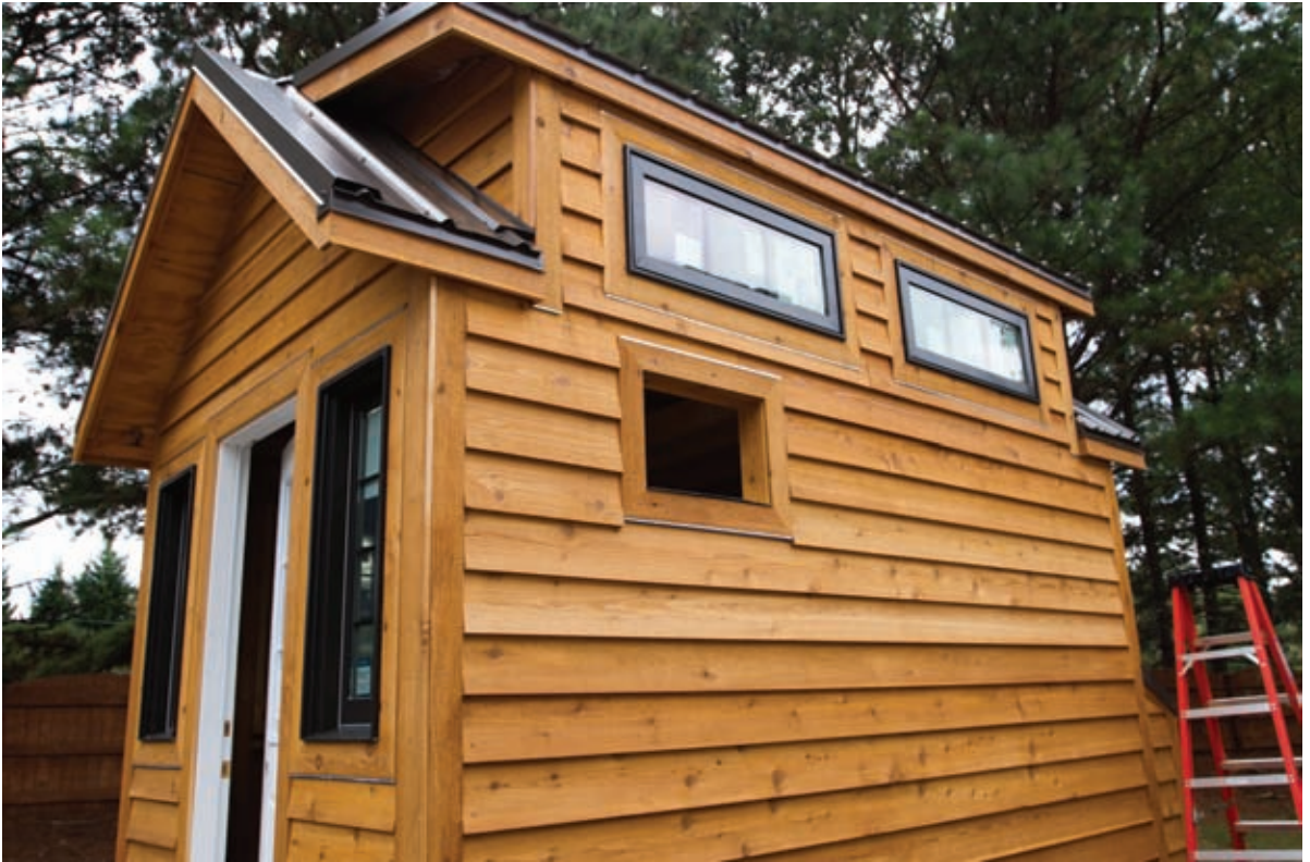
Siding Installed on the Side of the House
