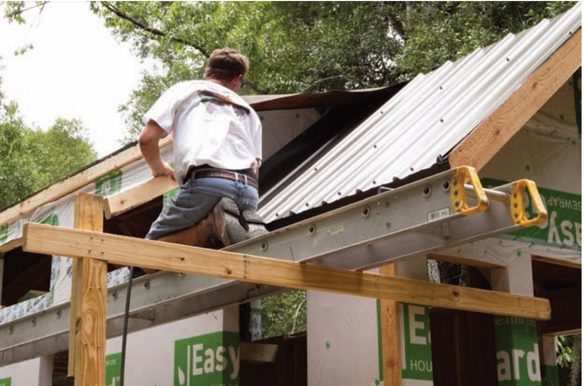
Side Wall Flashing Being Installed
