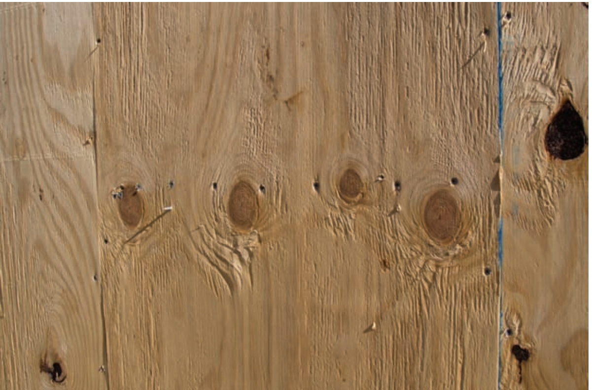
Wall Screwed from the Outside
