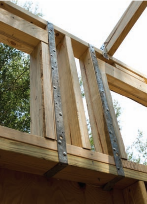
Strapping for Upper Walls
