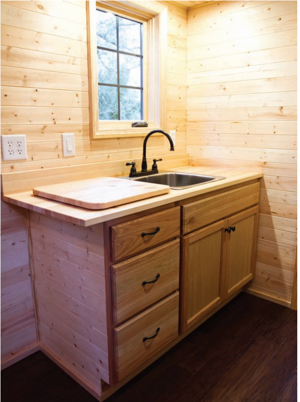
Pre-built Cabinets Installed
