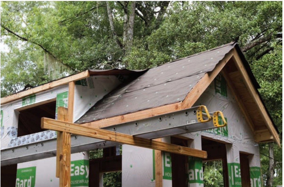
Tar Paper Installed
