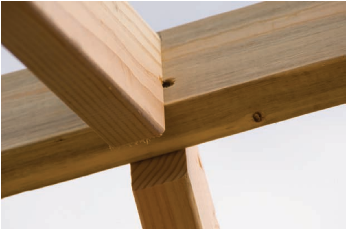
Rafters at Ridge Beam
